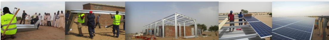
Construction and Commissioning of 3 Solar Photovoltaic microgrids in Chad on a Turn-key Basis, including techno-economic-social feasibility
